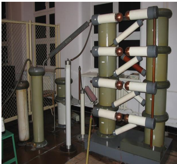
Fig. 3. Lightning surge generator station view.
