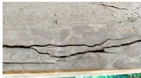
Fig.1. Structural Crack
