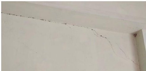
Fig.3. Joint Crack
