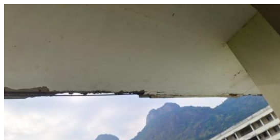
Fig. 2. Concrete Crack
