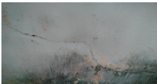
Fig. 4. Plaster Crack
