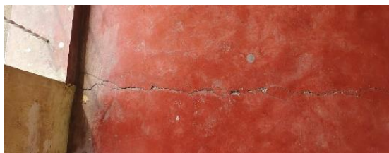
Fig.5. Floor Crack
