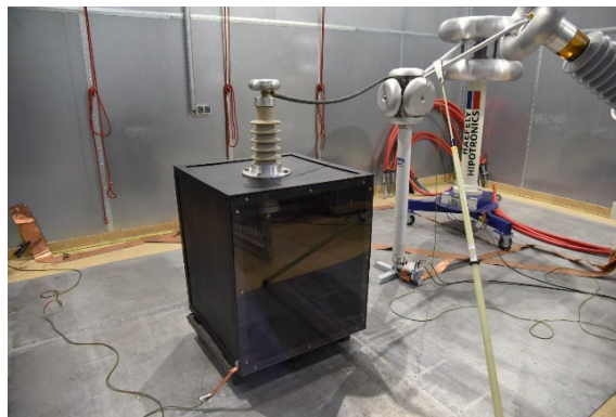
Fig. 1. The test object used during the measurements - a medium voltage switchgear model
