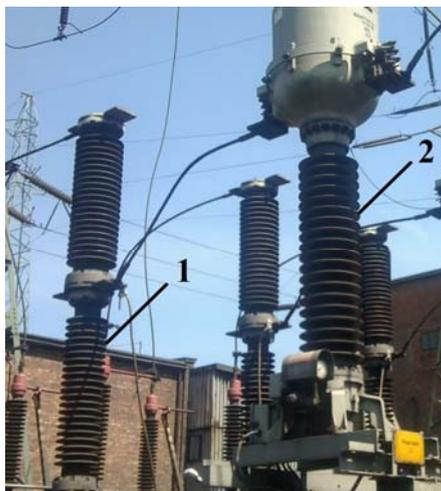
Fig.3. Porcelain housing (1) and silicone housing (2)
