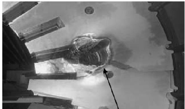
Fig. 1. An example of a broken stator core
