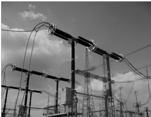
Fig.1. Overview of LTB 362-800 (T) E4 circuit-breaker by ABB
