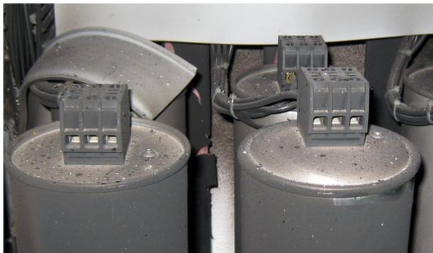
Fig. 10. Photograph of an example capacitor bank step after 5 years of operation
