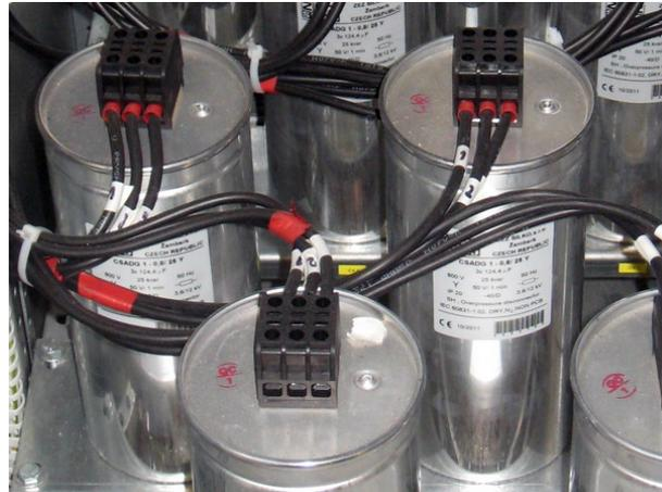
Fig. 7. Photograph of one of the steps of an example new capacitor bank
