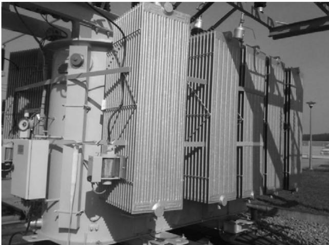
Fig.3. Transformer with radiators bound with cargo tapes
