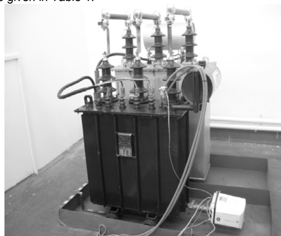
Fig.4. Measured transformer 30 kVA (black) and its power supply transformer (silver) in the laboratory
