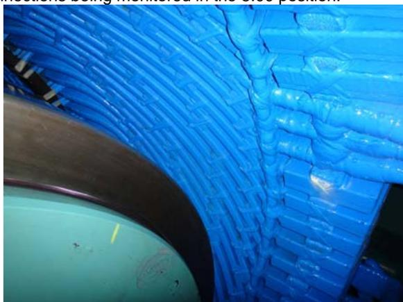
Fig. 2 Dusting on stator endwinding near 5:00 top connection
