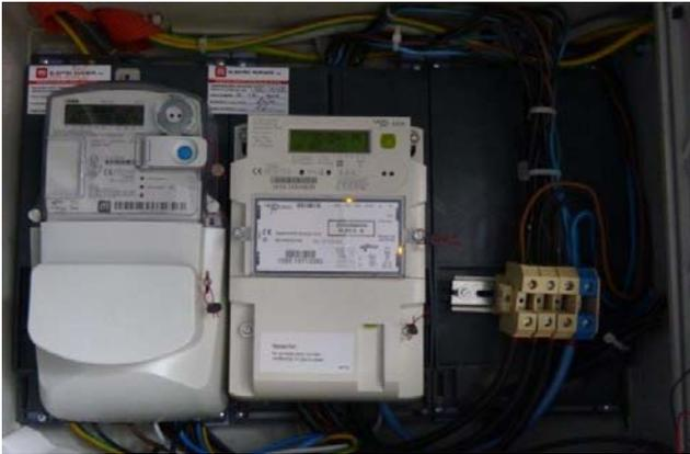
Fig.6. Pilot site – electric energy meter for electricity production and consumption
