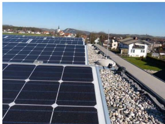
Fig.5. Pilot site - photovoltaic power plant with pyranometer
